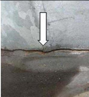
Close-up - crack near weld that joins the pole to its base plate
